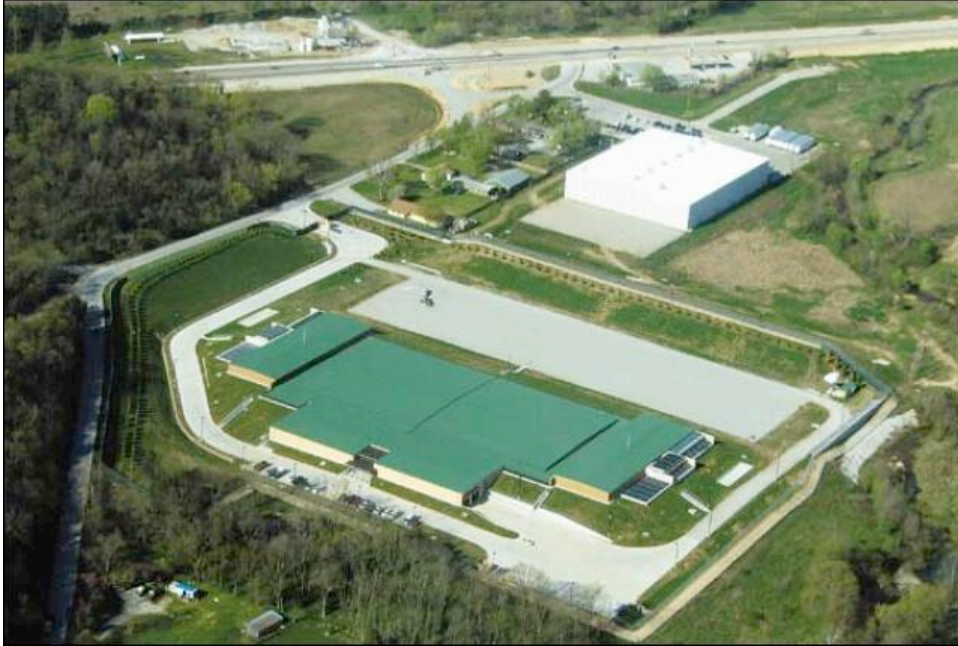
Figure 3: Wal-Mart Data Center in McDonald County is deemed so secret the county assessor was required to sign a non-disclosure statement before entering the site to determine property value. The photo was taken in 2004, when the center was nearly complete.
